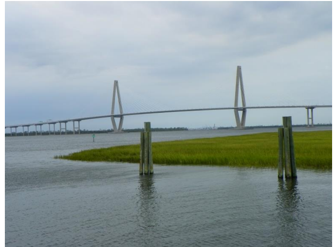
Bridge to Patriots Point
